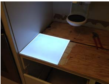
Figure 10 SLABlite tested, glued in place
